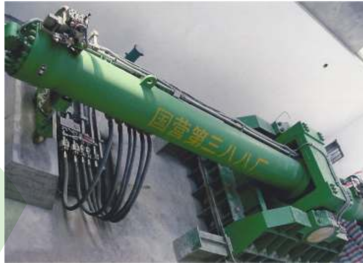
Three Gorges Dam (China), lock gate cylinders fitted with REGNIER INDUSTRIES's SENSO'R, linear stroke measurement system.
