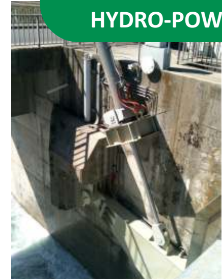
Manufacturing of a wide range of hydraulic cylinders and systems for radial gates dams.
